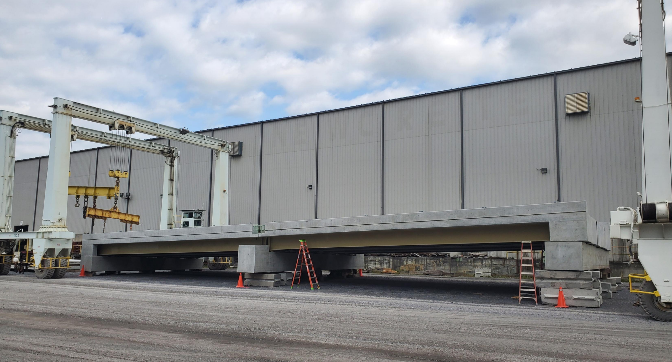
Complete Bridge "Dry Fit"
