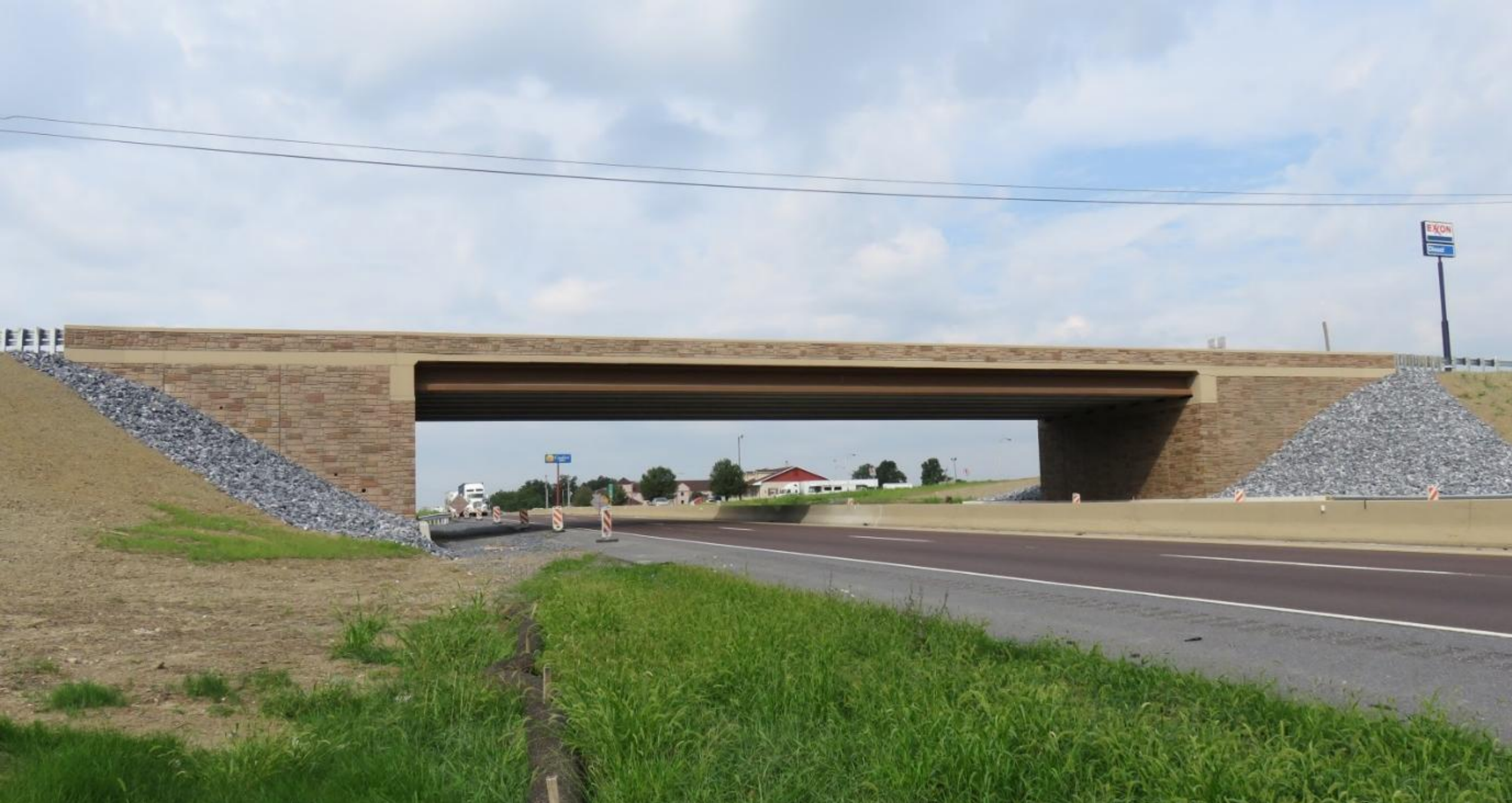
I-78 Underclearance Project – Berks County
