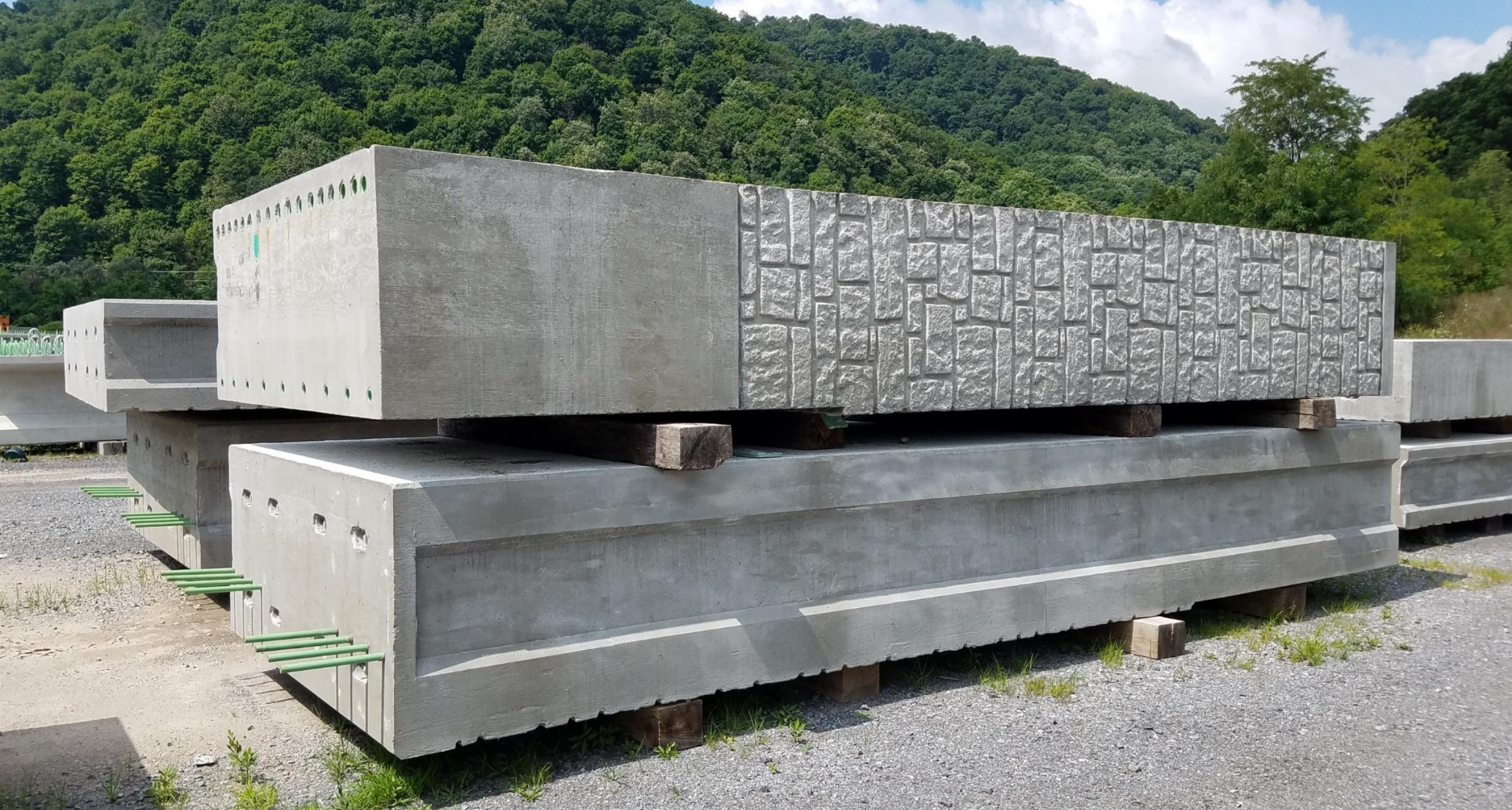
Finished abutment walls in the yard awaiting transport to the jobsite
