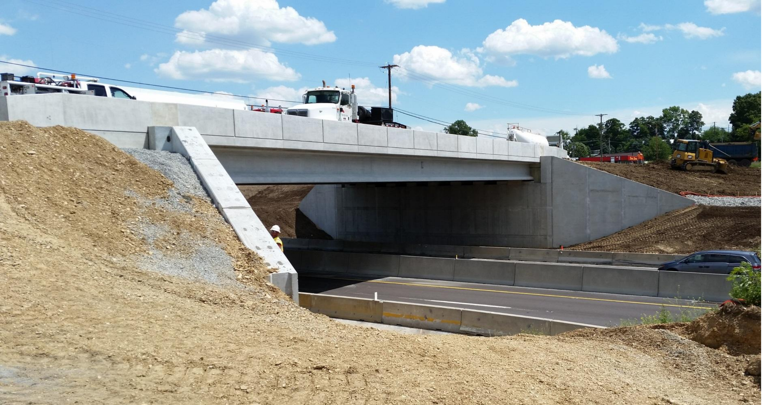
Bridge Constructed (Road close to Road open) in 30 Calendar Days
