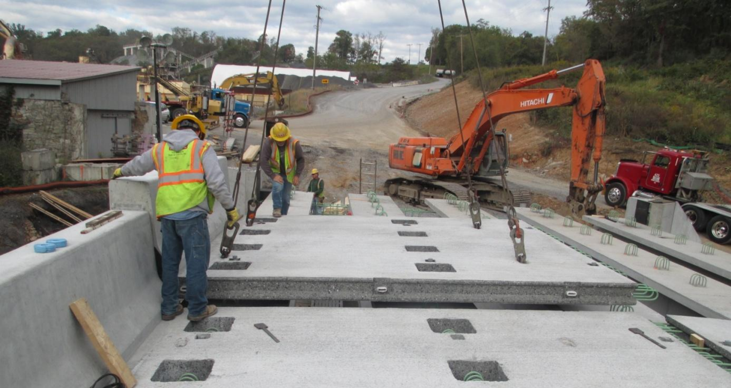
Full Depth Deck Panels with Integral Parapets on Bulb Tee Girders
