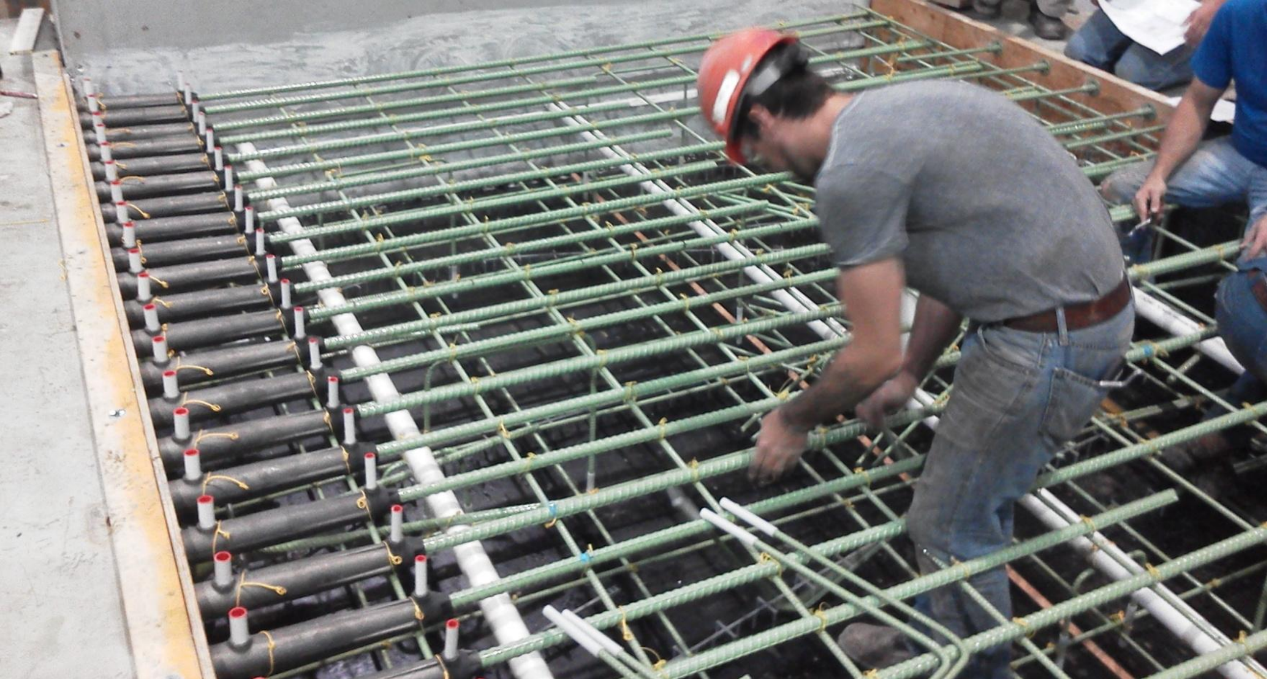
Match cast abutment wall – to column
