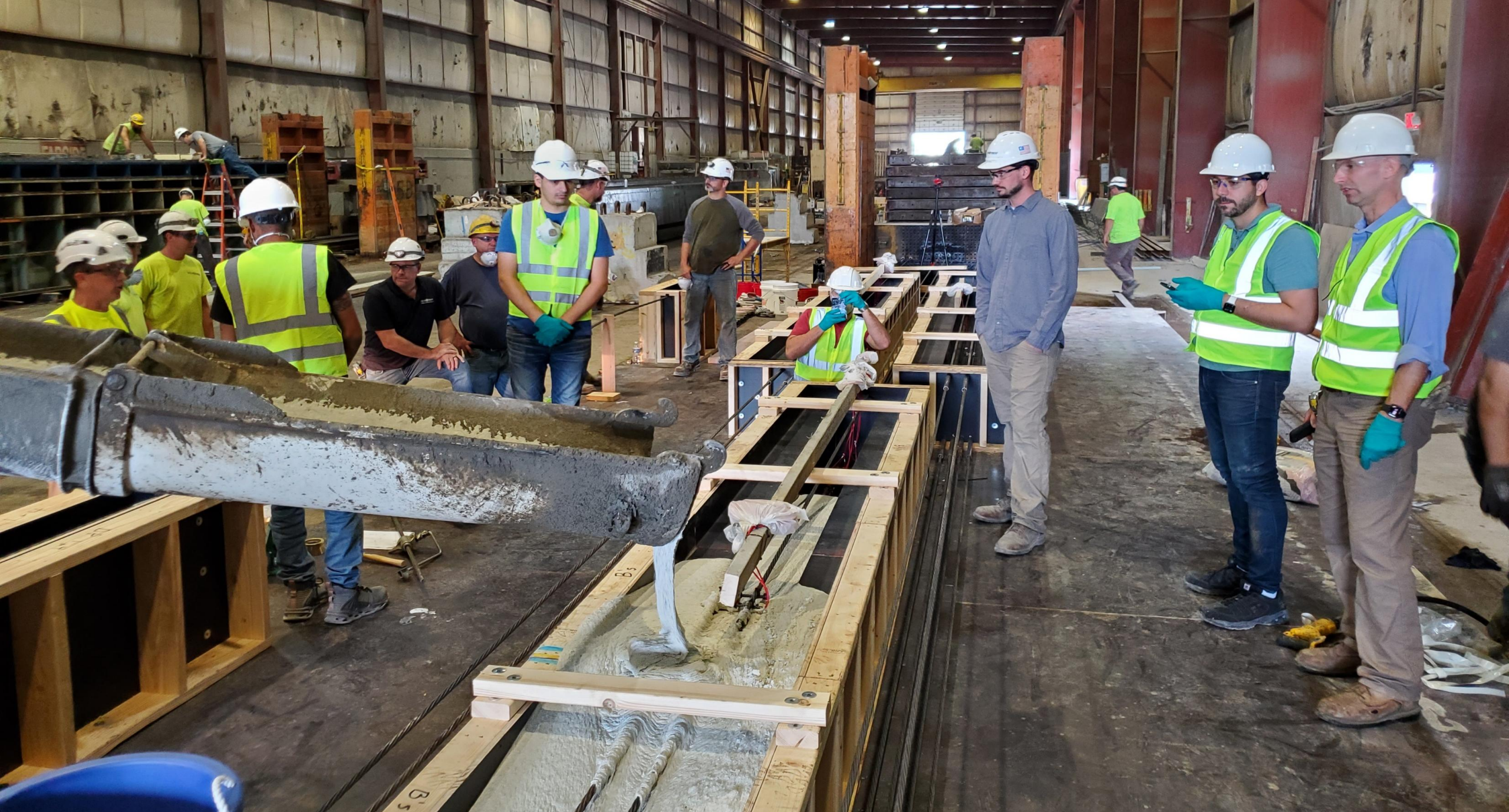
UHPC Federal Highway Research Project – September 2022
