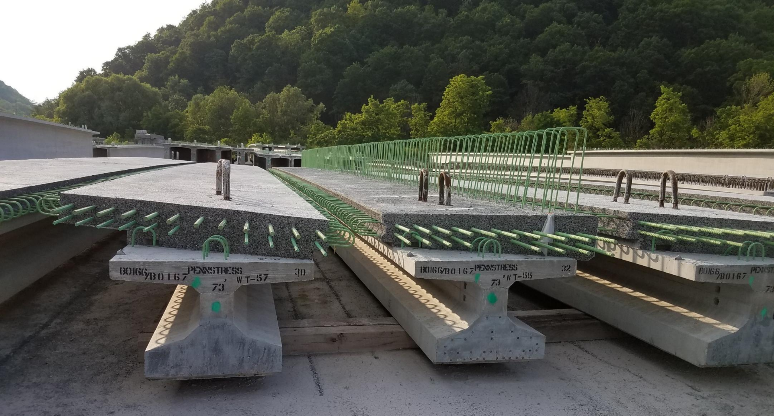
Modular decks on Bulb Tee Girders
