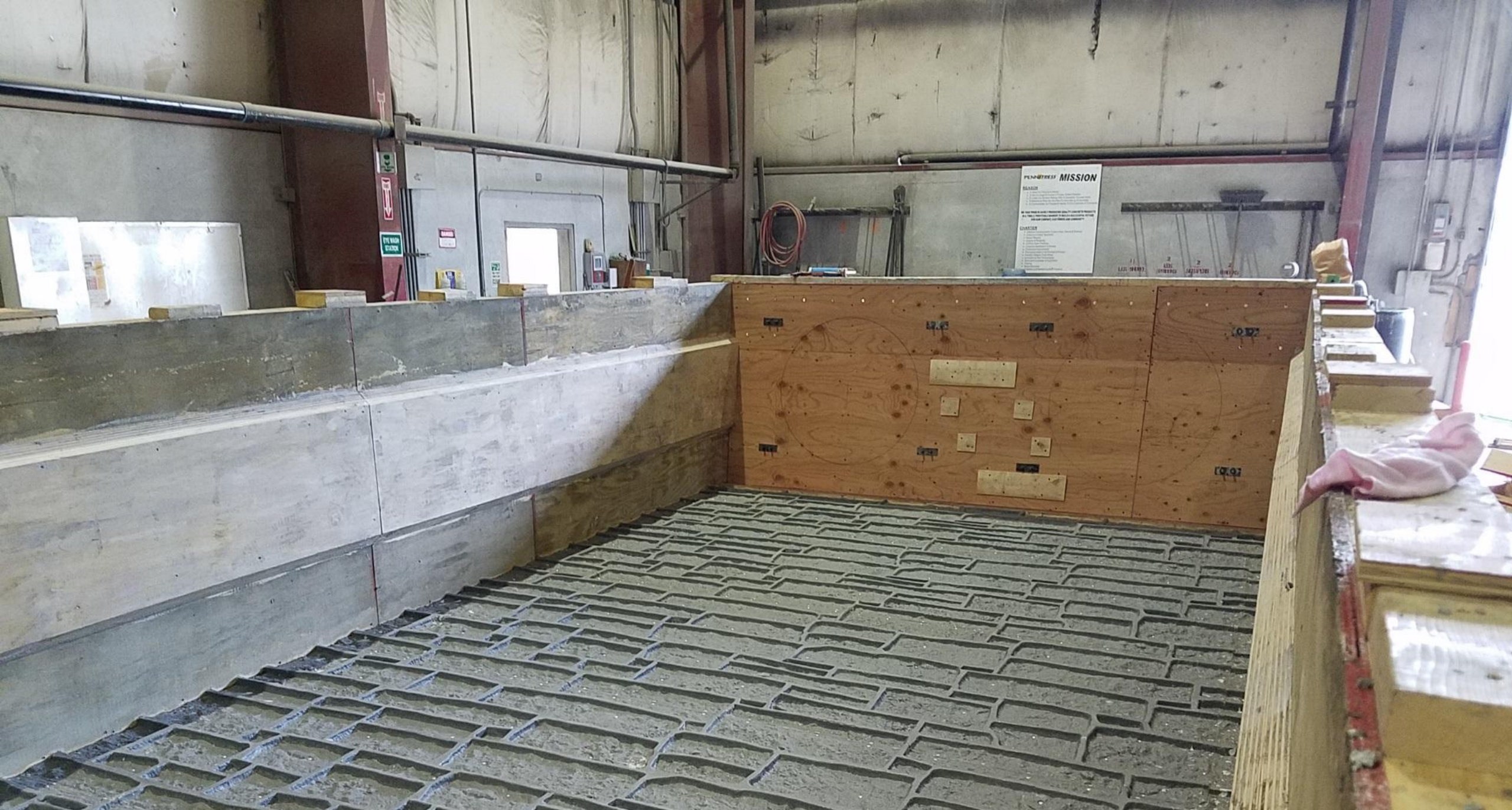
Abutment wall – Ashlar stone form liner
