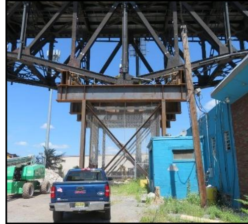
SUPPORT SYSTEM AT PIER 77 (EXISTING PIER REMOVED)
