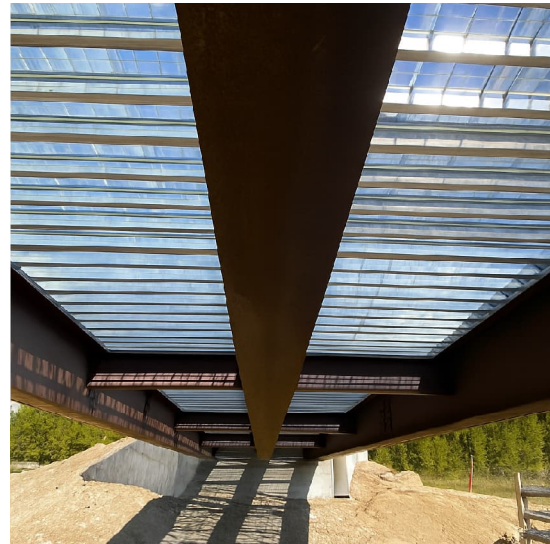
Installed ClearCast Decking on Big R Rolled Girder
