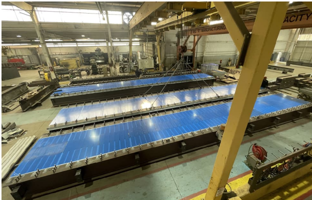
Big R Bridge Modules - Fabrication
