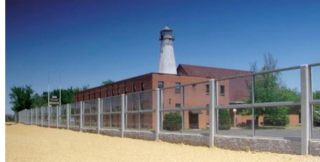
2009 Sound Barrier Installation (I-71 and Morse Road in Columbus, Ohio)
